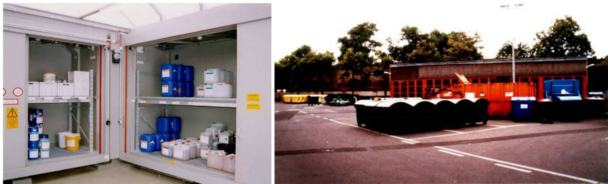
Pic: Hazardous waste and non-hazardous waste function area of a tertiary level hospital in Berlin
